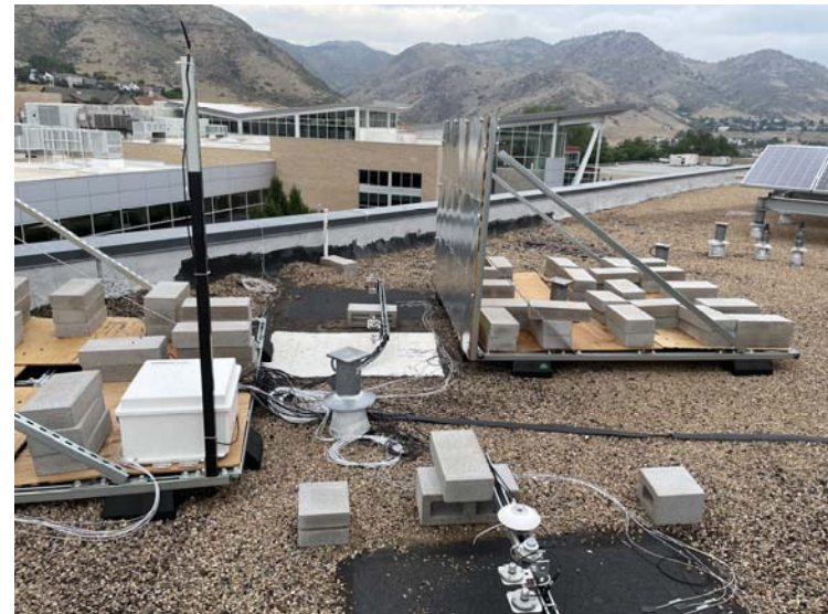
Roof membranes with adjacent vertical reflective panel surface
