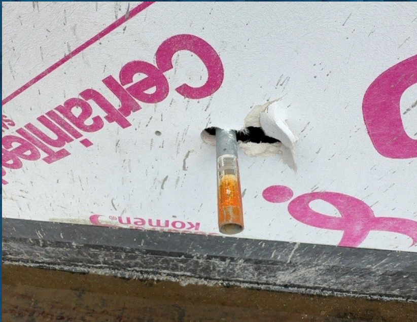
Pipe needs to be secured and accessible to detail
