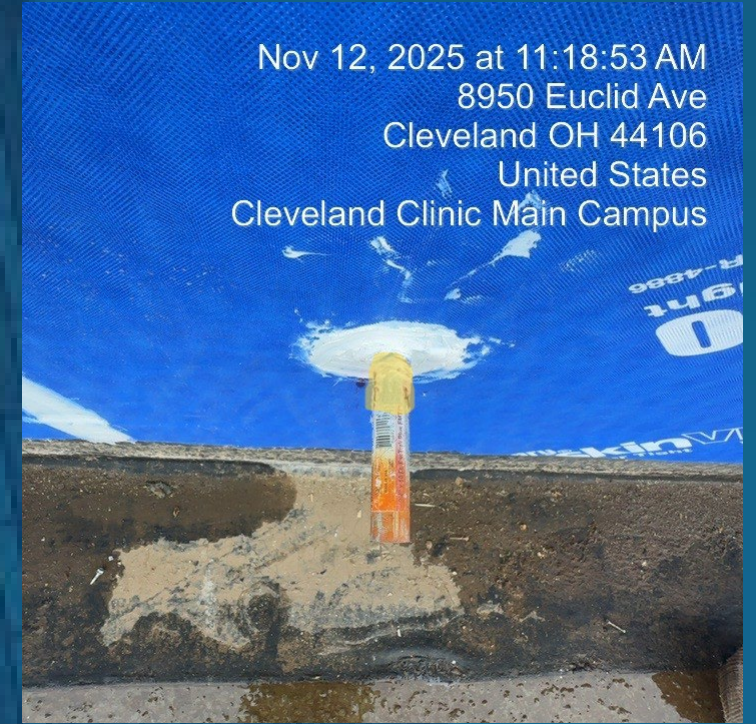
Seal onto the pipe, not just around it
