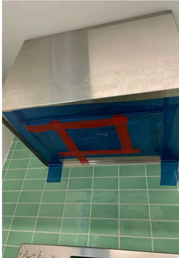
Kitchen exhaust sealed.
