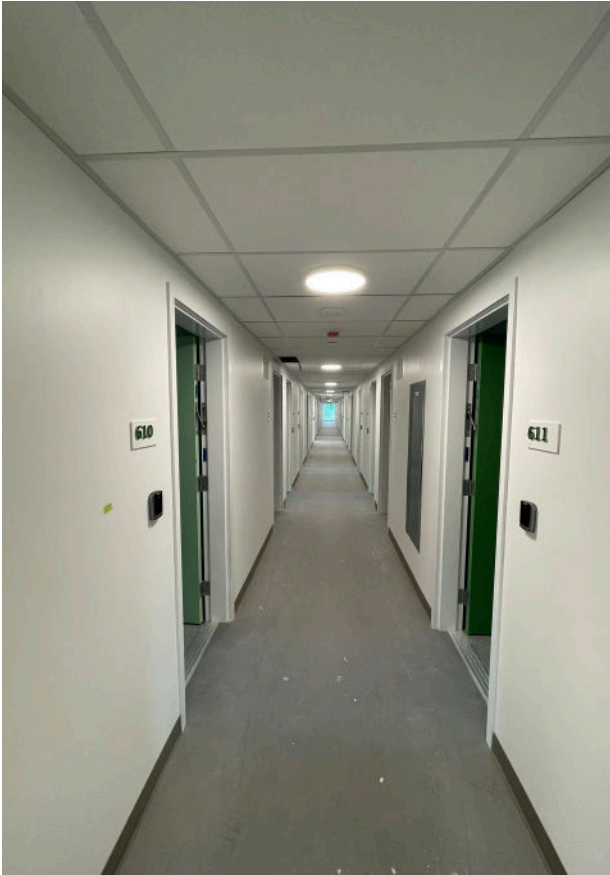
Interior doors propped open.
