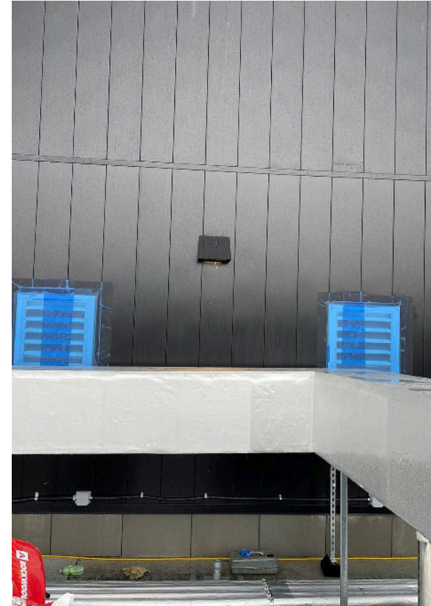
Exhaust fans sealed.
