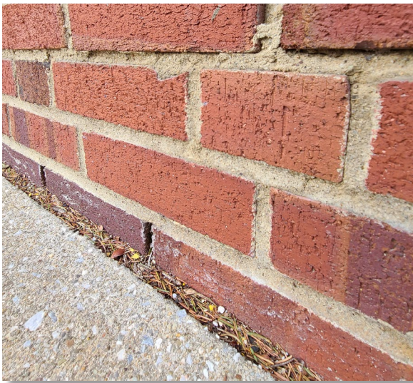
Open Head Joint (Weep)
