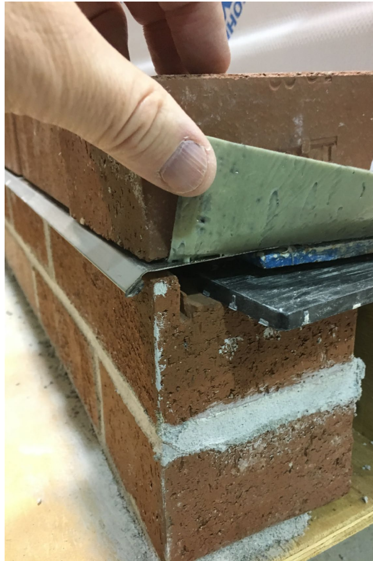
Through-Wall Flashing
