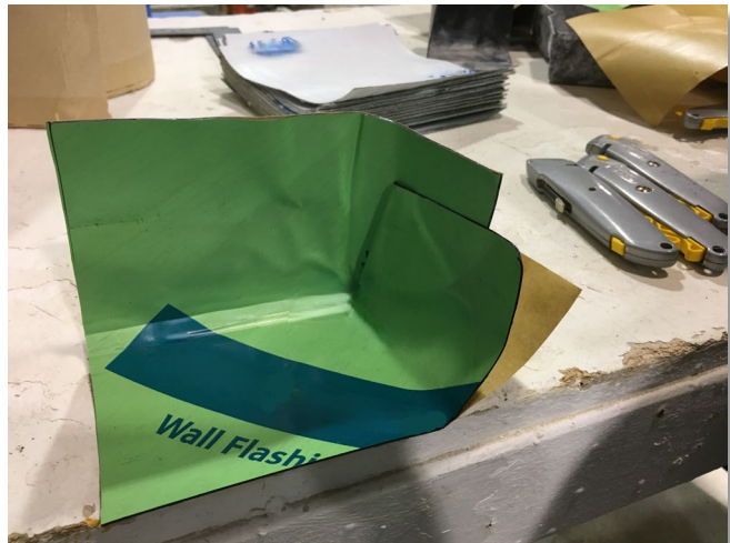
End Dam with Weep Vent
