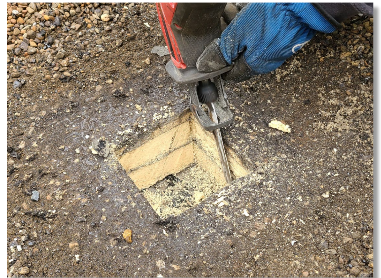
Roof Test Cuts
