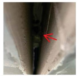
Unealed Splice Between Panels 10-09 and 10-10
