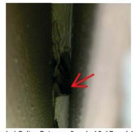
Unealed Splice Between Panels 10-17 and 10-18
