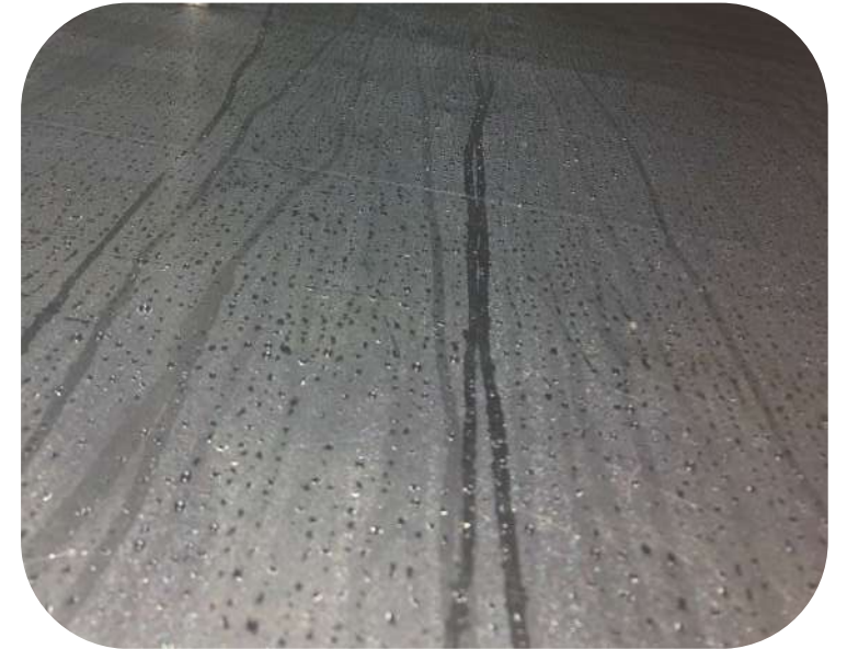
Condensation on mechanical duct
