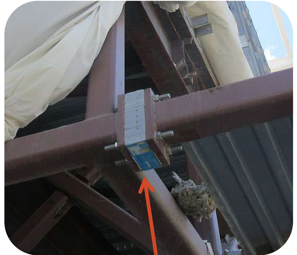
Thermal isolator pad at steel canopy support
