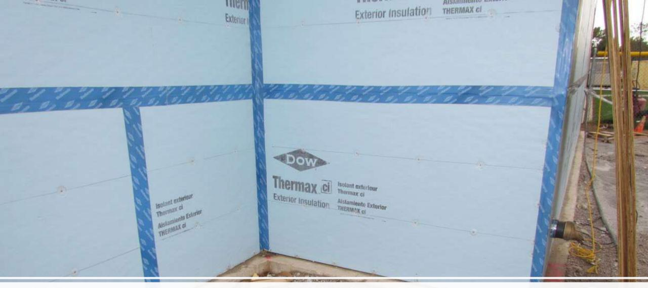
Air/Vapor Retarder - Insulation Board - Sealed
