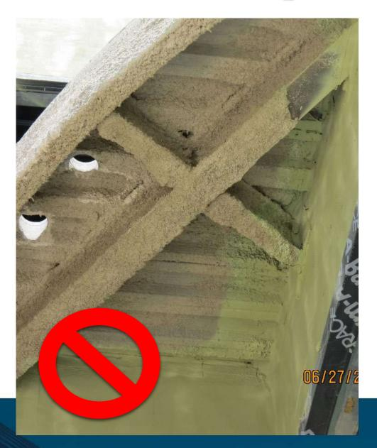
Unless allowable by the manufacturer and tested, SPF or AVB should not be on spray fireproofing
