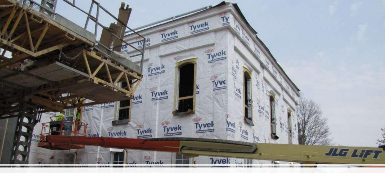
Air Barrier - Mechanically Fastened
