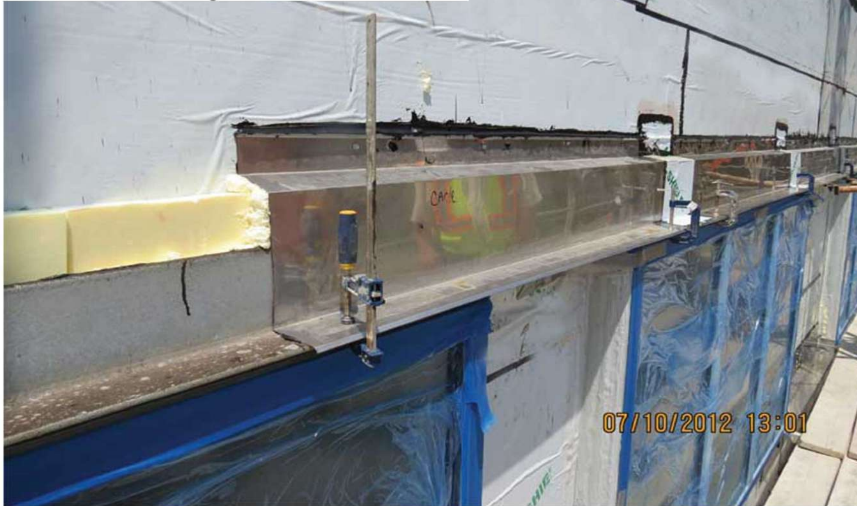
Image 3 of 3 - Creating a continuous air barrier from the wall to the shelf angle with a stainless steel flashing. The author also installed a spray polyurethane foam (SPF) solid under the stainless steel flashing to reduce the condensation potential under the flashing.
