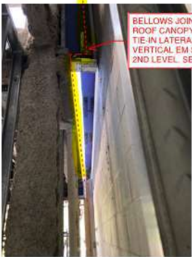
Location 2: Expansion joint at canopy
