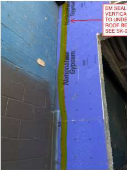
Location 3: Vertical expansion joint
