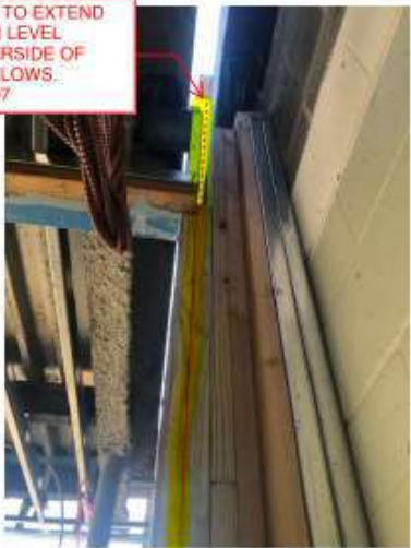
Location 1: Storefront expansion joint
