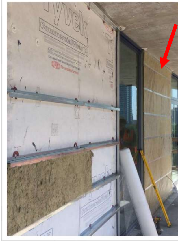
Exterior Insulation Attachment Mockup
