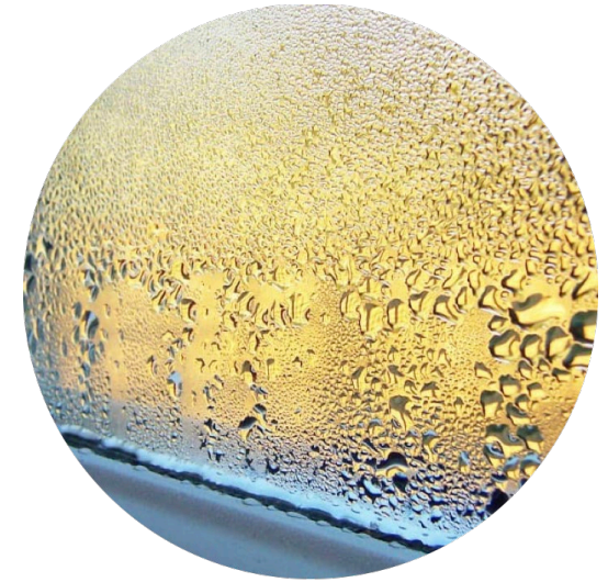
Condensation: Cold Surfaces
