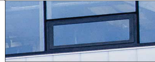
DETAIL OF THE CURTAIN WALL VENT ADAPTOR.
